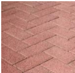
Pavés poreux (Source : Grand Lyon)
